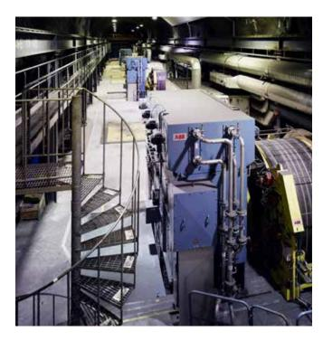
Certain ABB motors, whether variable speed drive (VSD) or direct online (DOL), boast rotors with heads weighing up to 130 tons and spanning four to eight meters in length. Enormous torque loads in cold conditions are brought to bear on the Ovakosourced shafts throughout their speed range.
